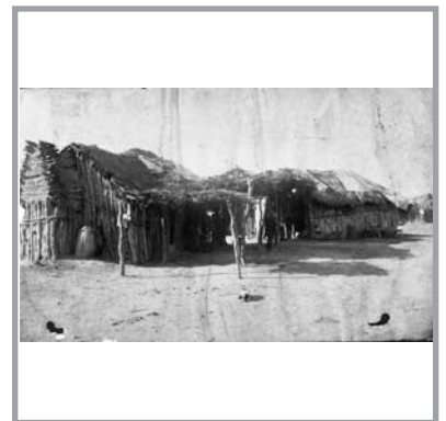
Exterior of the Sampson and Mary July residence, a jacal structure, Las Moras Village, a Black Seminole community adjacent to Fort Clark, Brackettville, c. 1905
